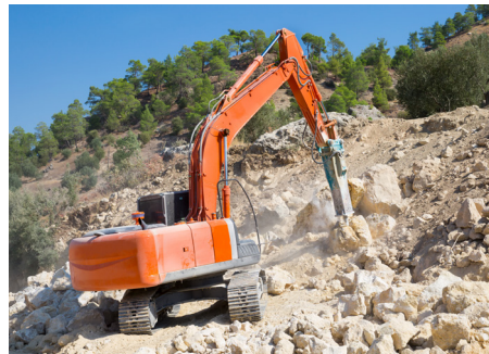
Excavator mounted with hydraulic breaker
